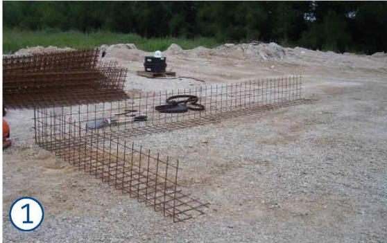
1 Preparation of base and first L-basket:
