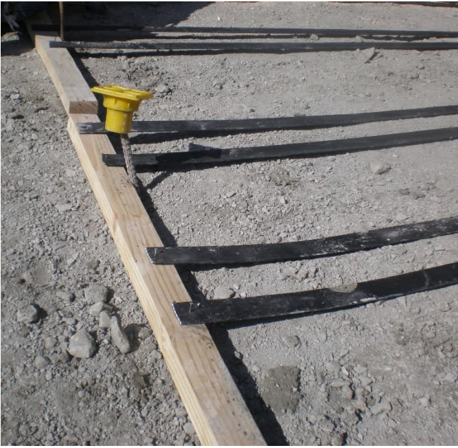
Figure 15: Lumber is held in place with a piece of rebar.
