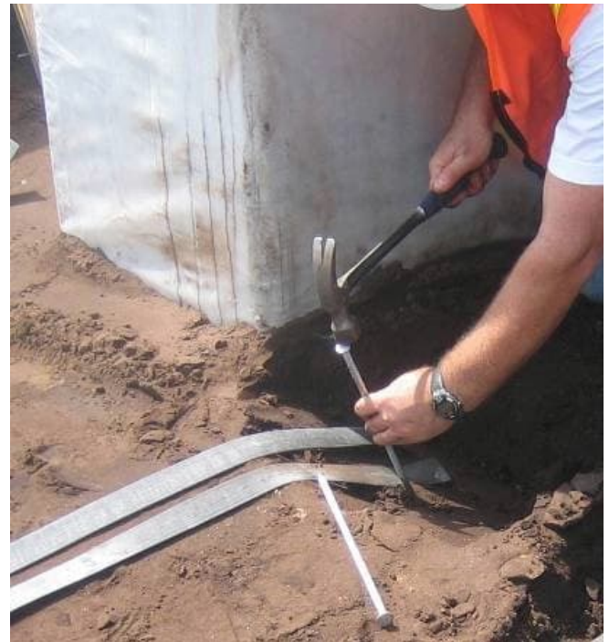
Figure 13: Securing the end of a GeoStrap in a hole with a stake.
