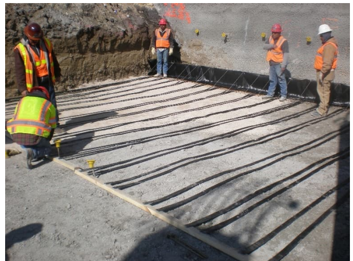
Figure 14: GeoStrap tensioned and secured to pieces of lumber.
