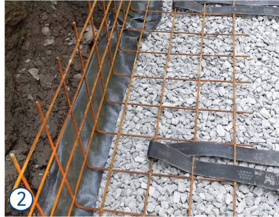
2 Installation of the first GeoStrap course:
