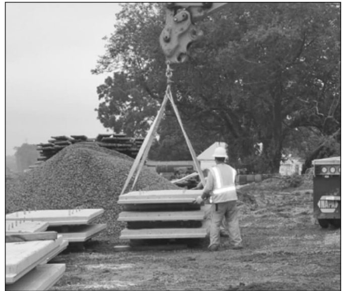
Figure 7: Lifting devices for handling individual panels.
