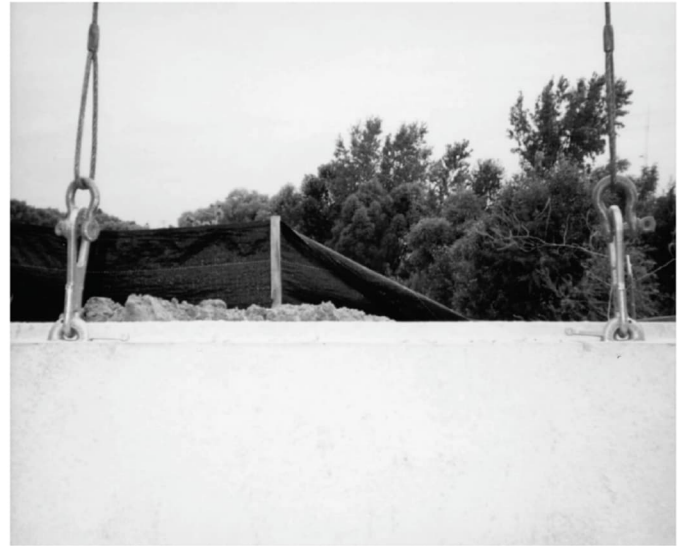
Figure 6: Lifting devices for handling individual panels.
