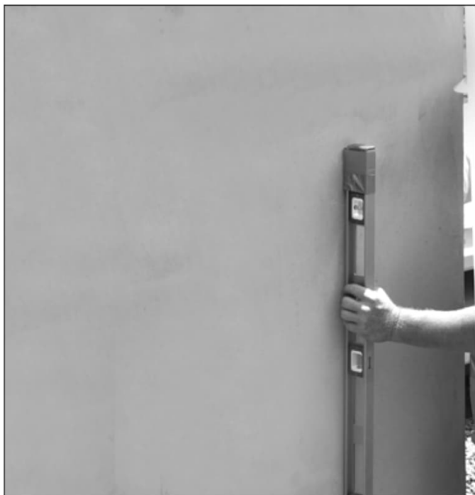
Figure 18: Set panel batter
