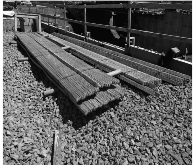
Figure 9: Reinforcing strip bundles stored on site.
