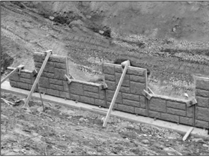
Figure 22: Braced initial course of panels.
