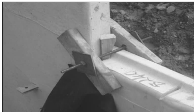
Figure 21: Panels secured with a clamp.
