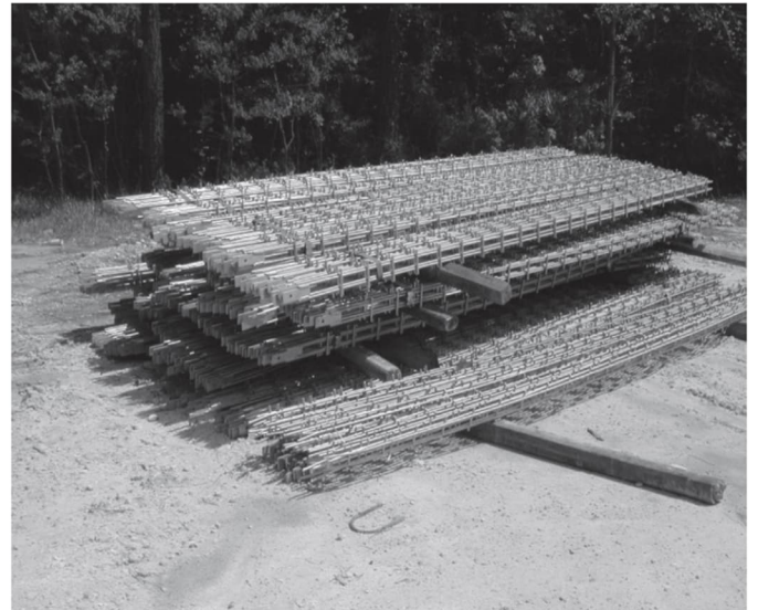
Figure 10: HA Ladder reinforcing strips stored on site.
