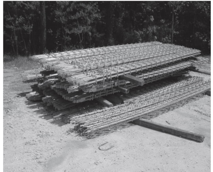
Figure 9: HA Ladder reinforcing strips stored on site.
