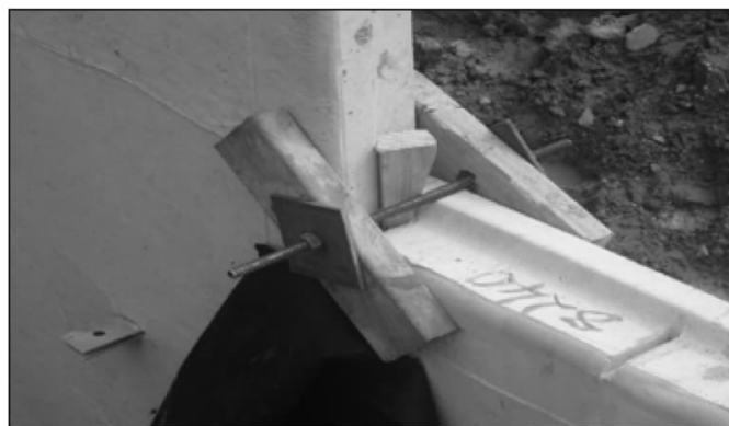
Figure 20: Panels secured with a clamp.
