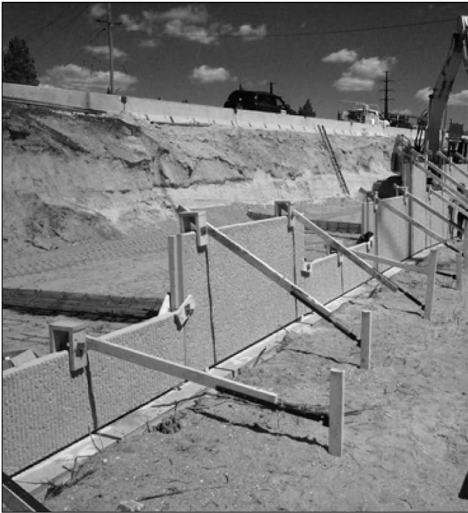
Figure 21: Braced initial course of panels.
