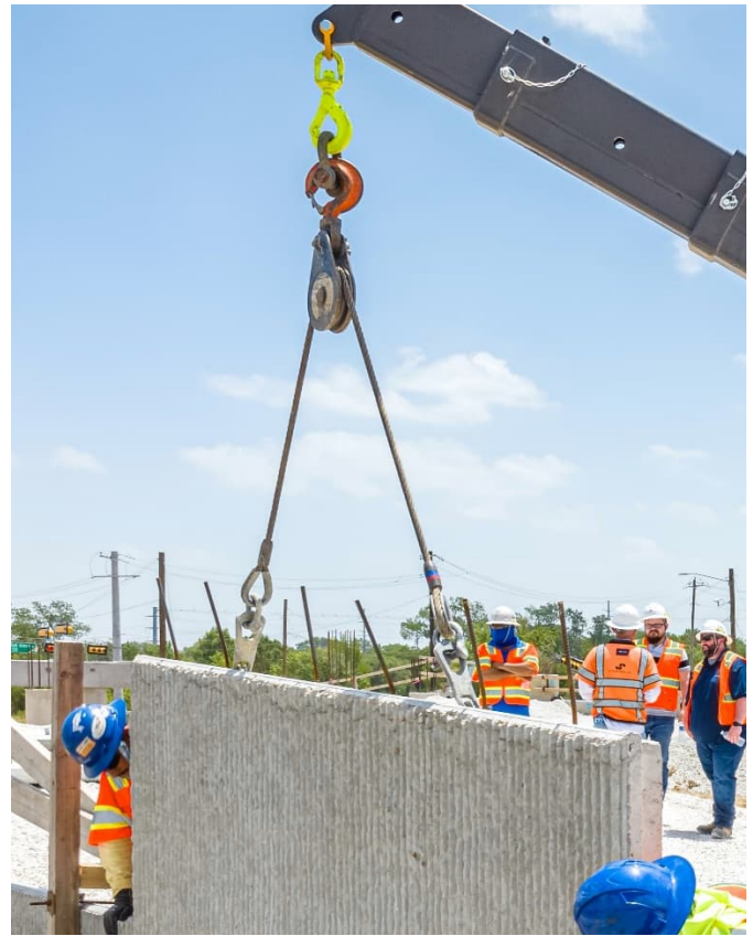
Figure 6: Lifting devices for handling individual panels.
