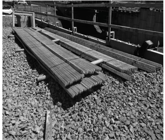
Figure 8: Reinforcing strip bundles stored on site.
