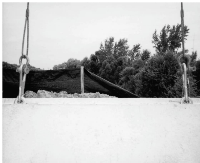
Figure 6: Lifting devices for handling individual panels.
