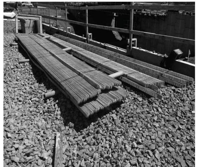
Figure 9: Reinforcing strip bundles stored on site.
