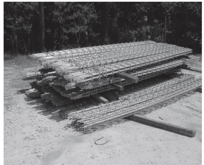
Figure 10: HA Ladder reinforcing strips stored on site.
