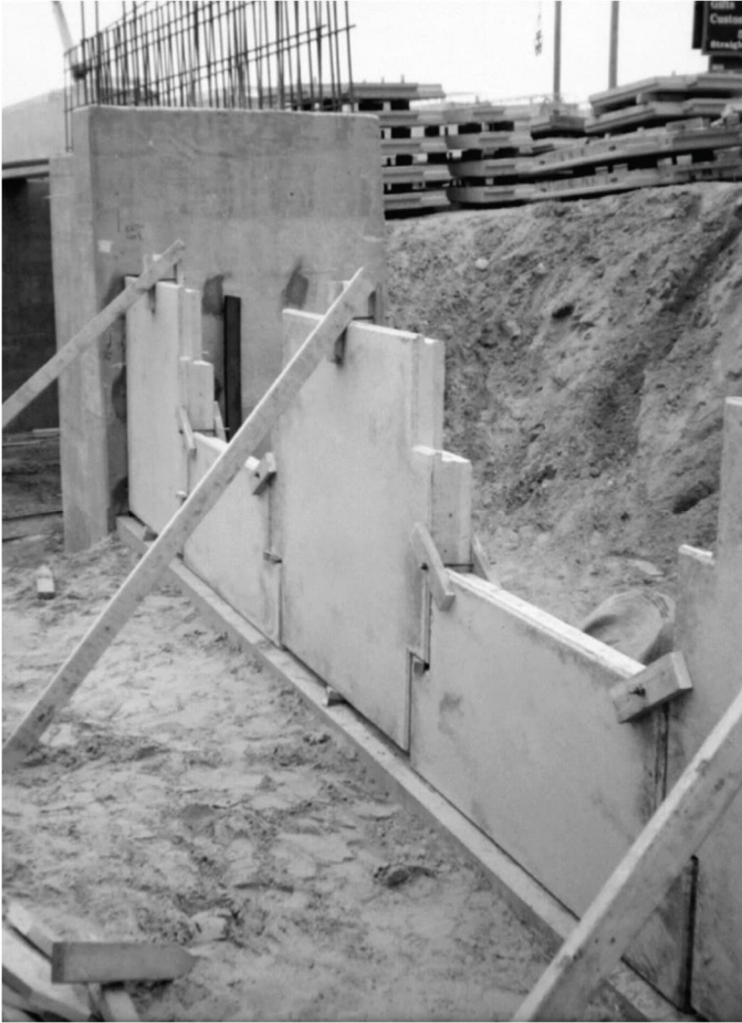
Figure 22: Braced initial course of panels.
