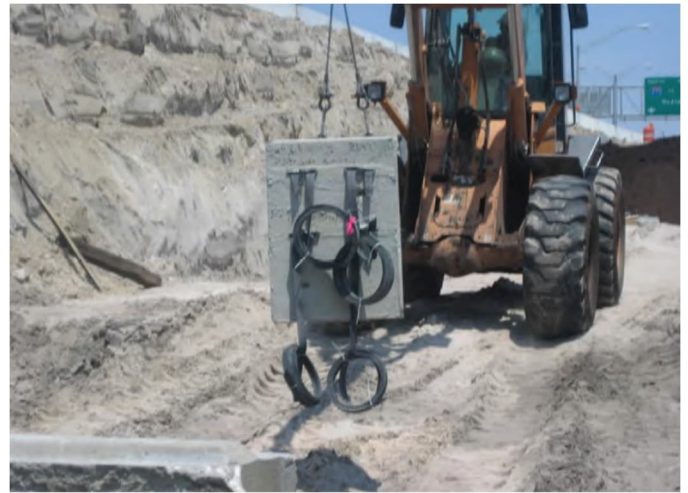
Figure 7: Lifting devices for handling individual panels.
