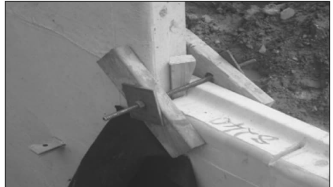
Figure 21: Panels secured with a clamp.
