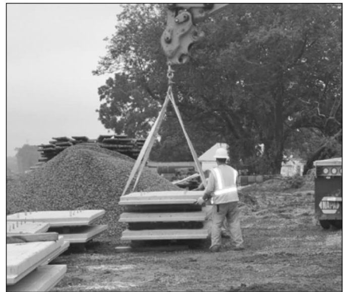
Figure 8: Lifting devices for handling individual panels.
