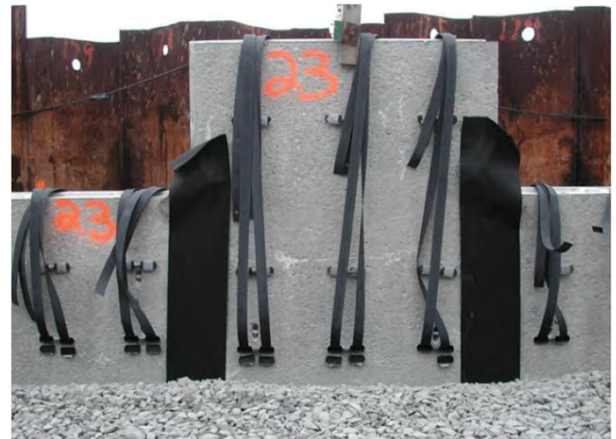
Figure 2: Square panel with GeoStrap and geotextile awaiting backfill
