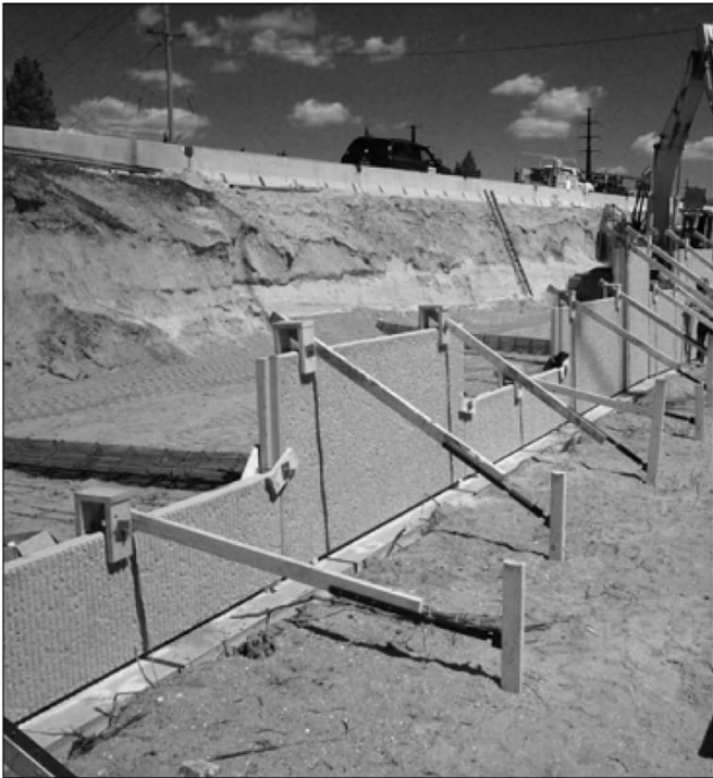
Figure 22: Braced initial course of panels (Rectangular panel type shown with two braces per A panel).
