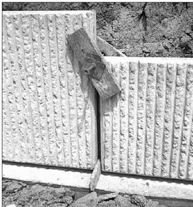
Figure 15: Panels braced with wooden clamp and spacer
